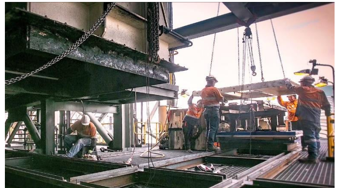
Old Plates removed and railed out using a track mounted hydraulic lifting table.
